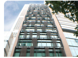
Located at 55 Market Street At the heart of CBD, Raffles Place
